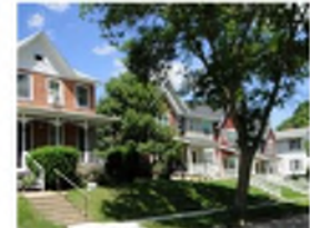
Orient a building to face the street, where this is an established component of the context's character.
